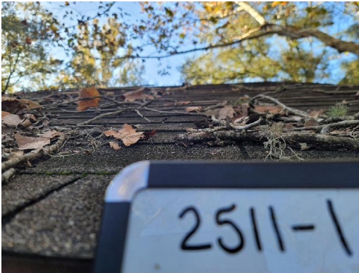
2511-1 Asphalt Shingle Typical Exterior Roof
